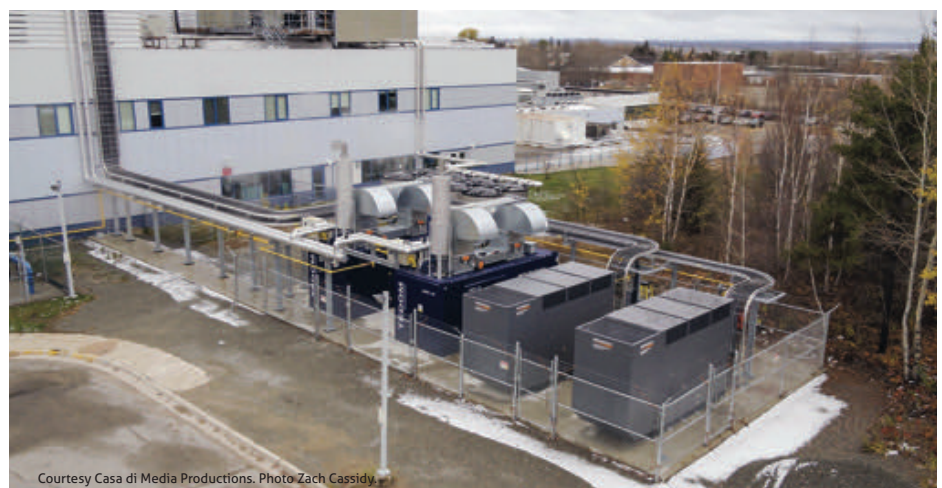
The completed CHP installation at Timmins and District Hospital.
